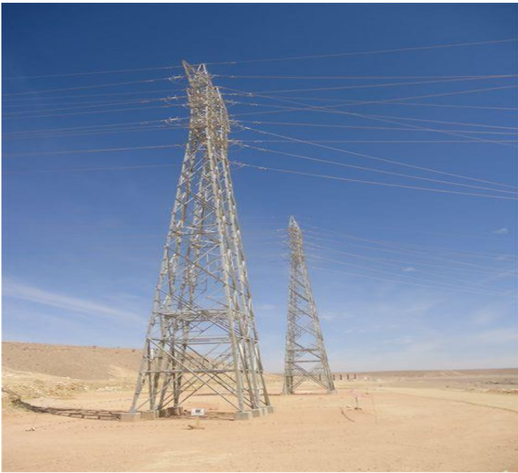
33KV OVERHEAD TRANSMISSION LINE TOTAL; YEMEN -2011-2012
