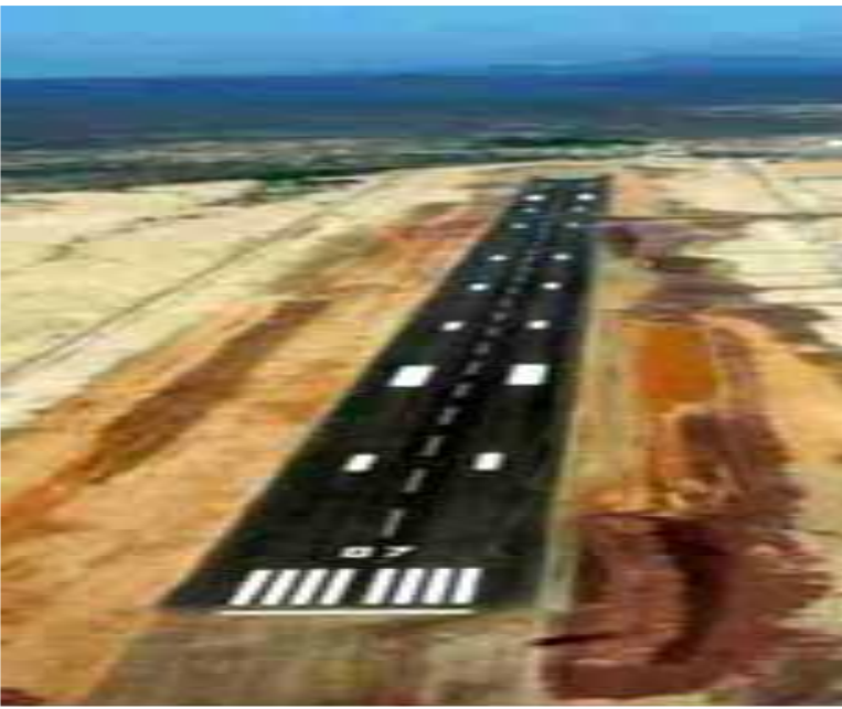
BALHAF YLNG PLANT RUNWAY CONSTRUCUTION YEMEN; 2006
